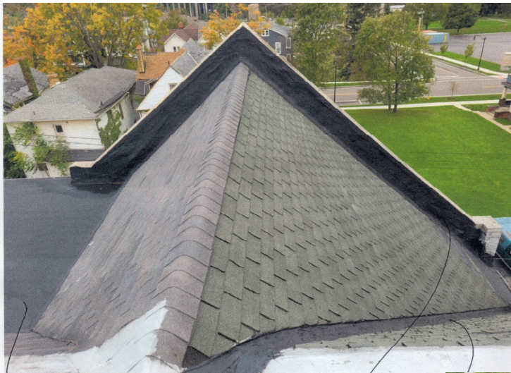
New roof sections with parapet repair with new flashing.
